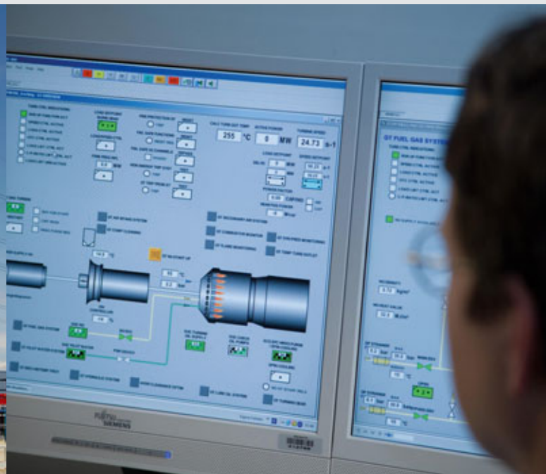
VM600 data are used for turbine monitoring (copyright Siemens AG)
