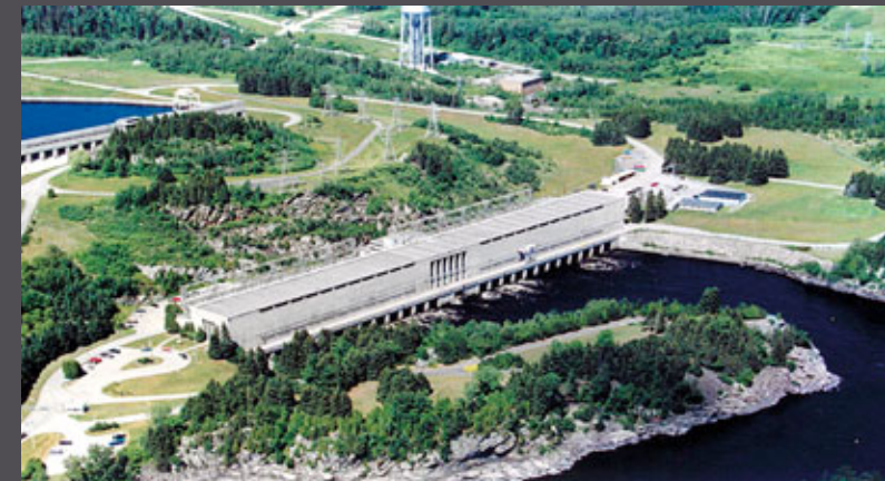
Shipshaw HPP (courtesy of Alcan Canada)
